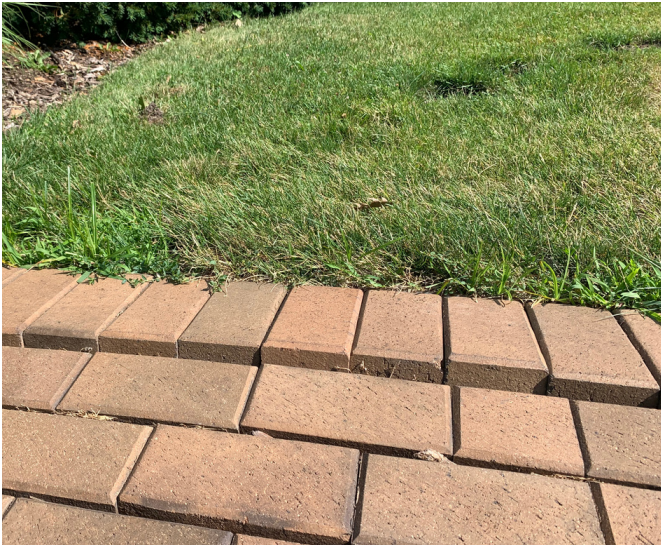
In the Judith A. Delapa Perennial Gardens, outer bricks 'rolling', causing a significant trip hazard (left) are being repaired with concrete curbs that will prevent the outer bricks from moving (right).
